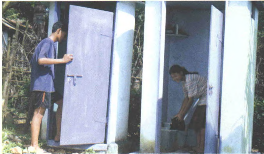
Two examples of pour-flush composting toilets
