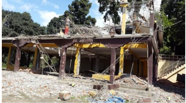
Kopan's beloved Chenrezig gompa undergoing preliminary demolition before rebuilding begins.
