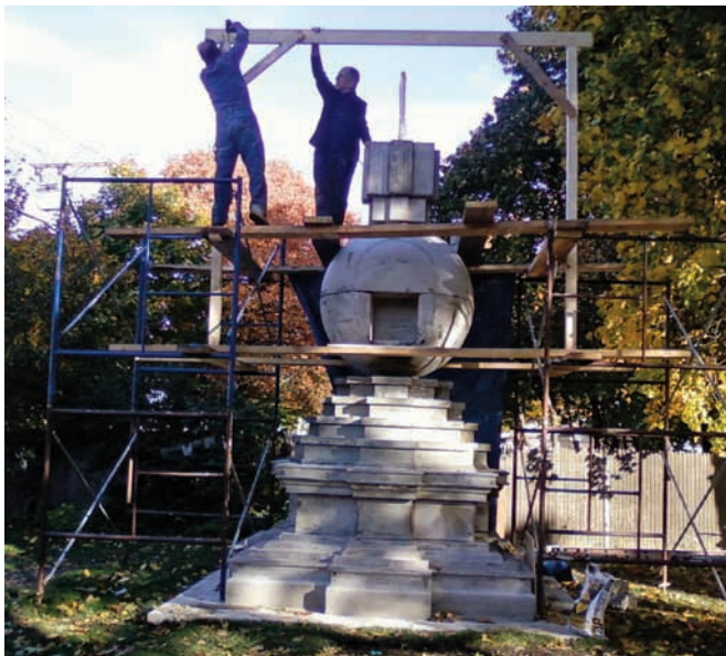
Construction of the Kalachakra stupa at Kurukulla Center
