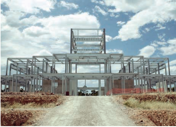
Construction of the Great Stupa begins
