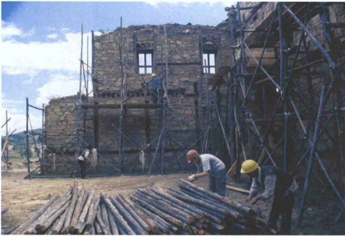
The crew assembles the timber scaffolding for work in the main building
