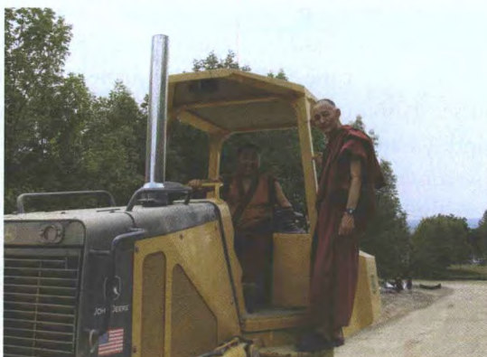
Namgyal monks get their hands dirty at the construction site.
