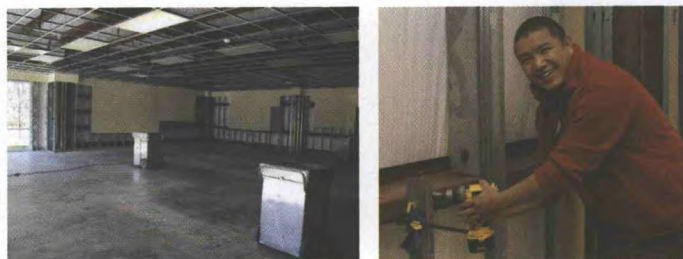
From this ... and thanks to Geshe Gelek's input ...
