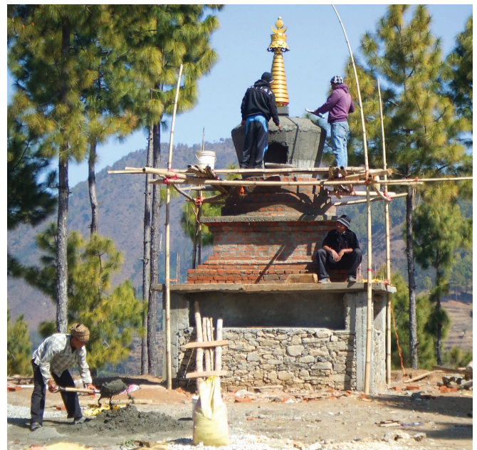
Stupa construction in Nuwakot, Nepal. Photo courtesy of Losang Namgyal Rinpoche.
